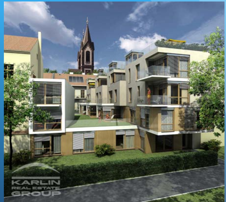
Social Housing Karlin, Praha CR Architect: Safer – Hajek Architects
