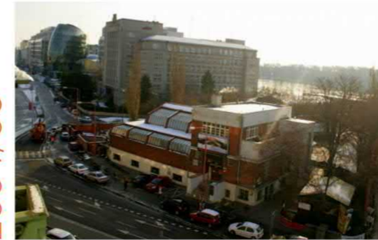
Large restoration of the building.
